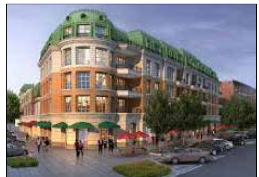
Figure 17: Mixed use building with mansard roof
