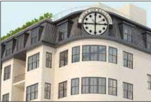
Figure 18: Mansard roof typ.
