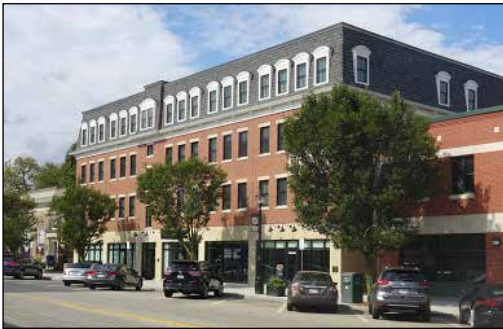
Figure 13: Mixed Use Building with Mansard Roof
